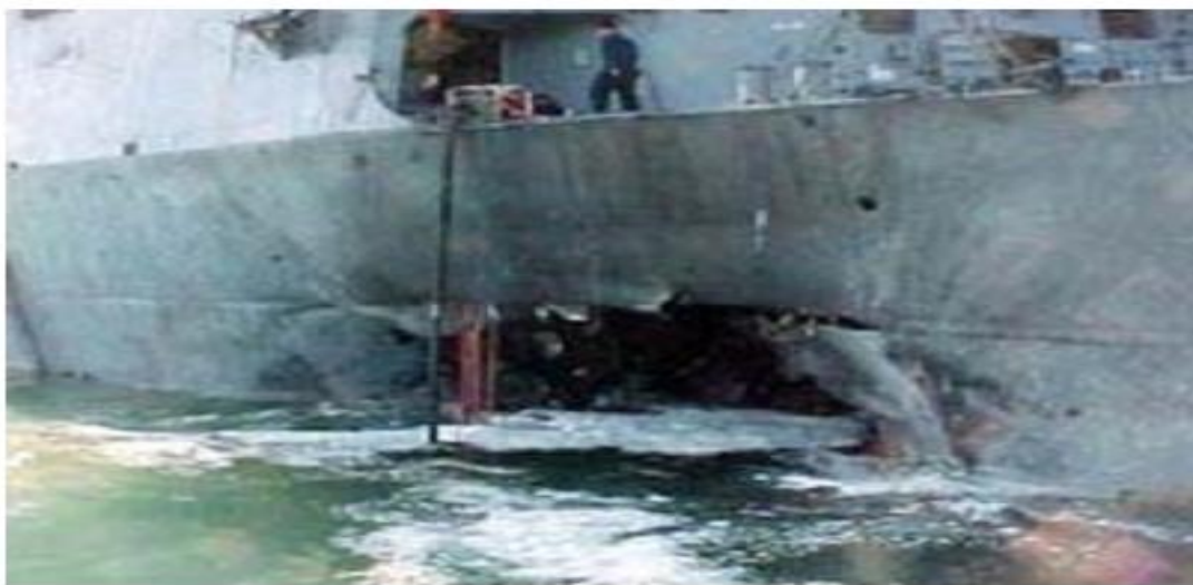
Figure 6.2.4: Close-Up of Hole in Hull of Cole
